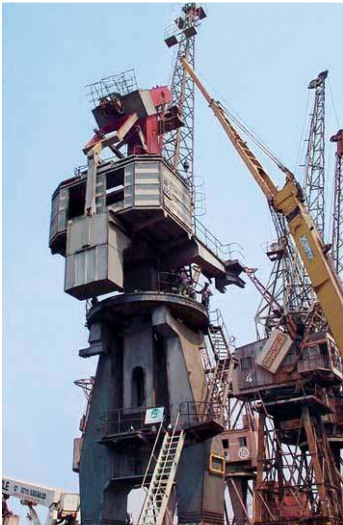
↑ Alter Kran in Porto de Luanda/Angola
